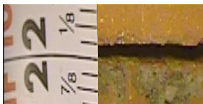
Interior Chimney photo taken by a Chim-Scan®
