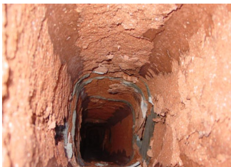
Exhausting high efficiency gas can erode liners
